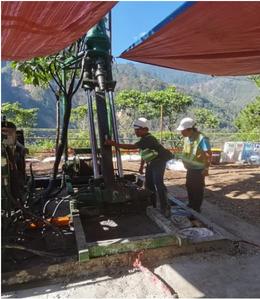
Image 1: Final incline check at MCB-034
